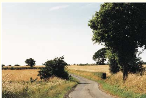
Garswood Old Road
