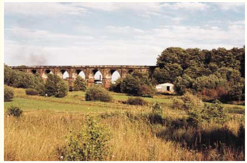
George Stephenson's Sankey Viaduct
