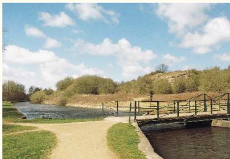
Swing Bridge over the St Helens Canal
