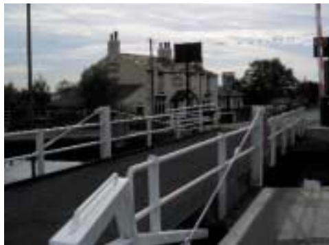
The Swing Bridge at Bells Lane
