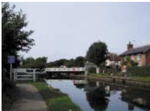
The bridge at Hall Lane
